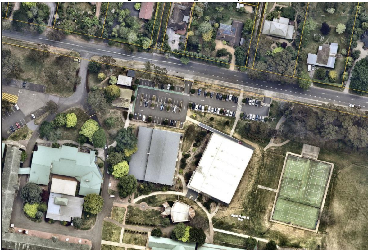
Figure 2: Inset Aerial Image (Nearmap)
