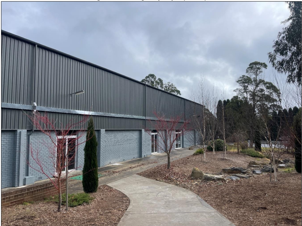
Figure 8: Eastern elevation of McGrath Hall as existing (Author)
